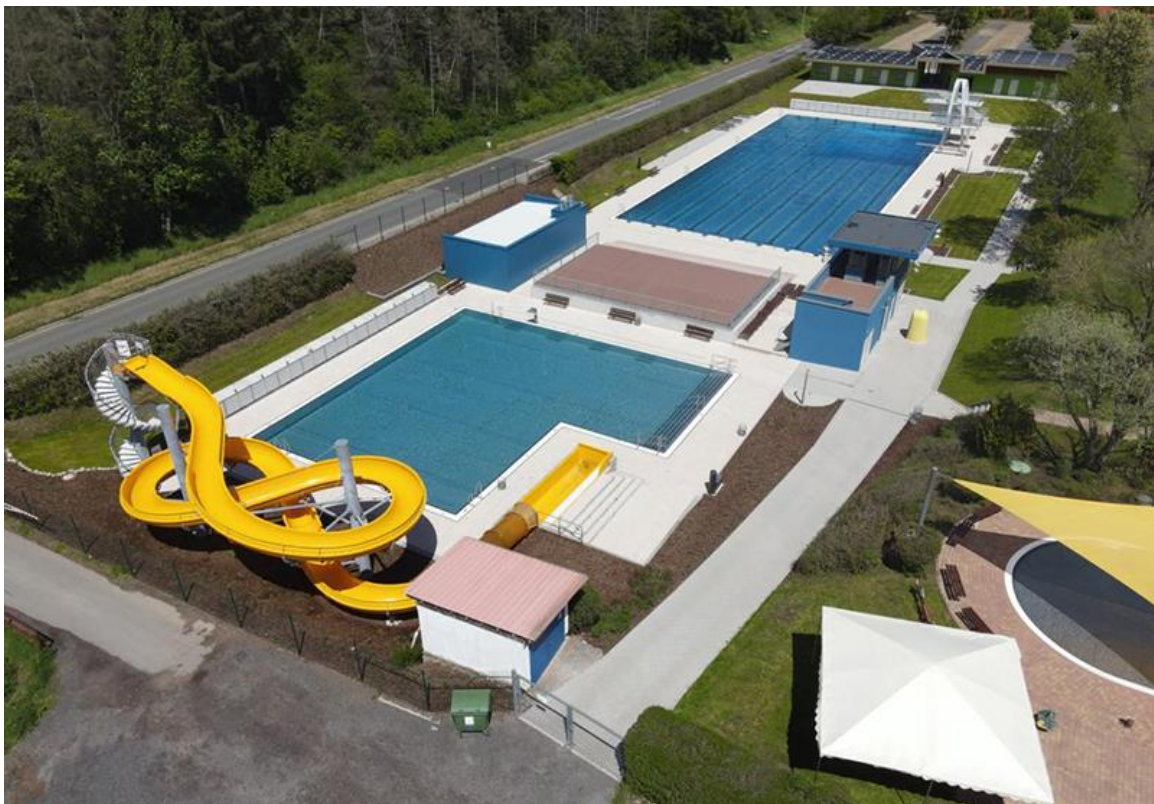
Picture: Verbandsgemeindewerke Winnweiler
