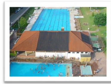
Aerial view of the outdoor swimming pool before the renovation measures
